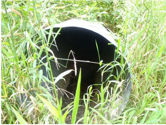
Photo 19: Culvert under Middleblock Road
