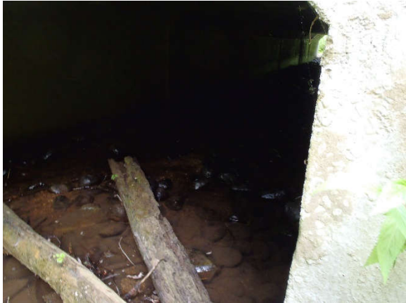
Photo 8: Culvert under road
