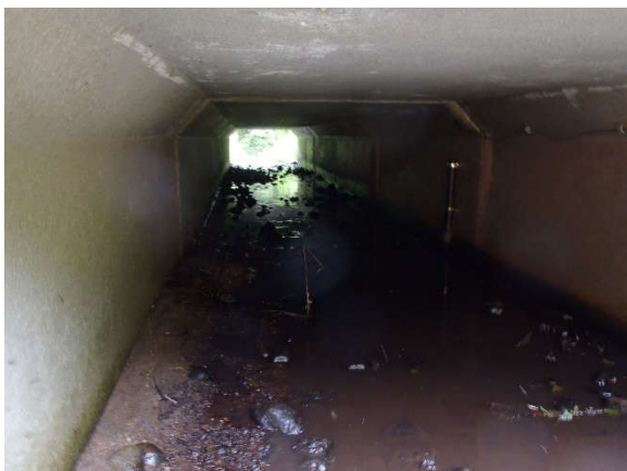
Photo 9: Second culvert under road
