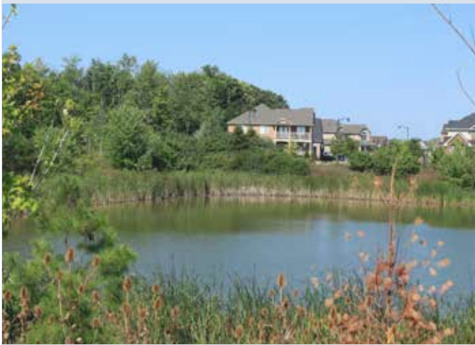
Image example showing dwellings flanking onto a SWMP, emphasizing the pond as a key feature of the community.
