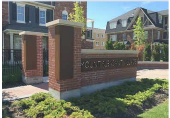
Image example of entry features used to reinforce the identity of the community through material selection and signage.
