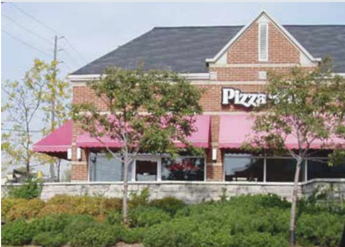
Image example of drive-through facility which offers ample landscaping and whose drive-through lanes are oriented away from immediate public view.
