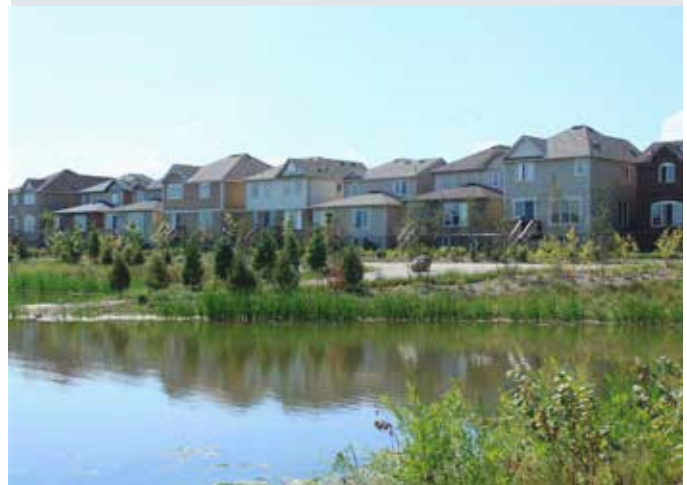
Image examples of upgraded rear elevations that back onto parks and open spaces and that are highly visible to the public.
