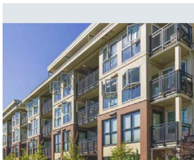
Image example of high density mid-rise apartment building with private open space amenity areas to enhance the private living environment.
