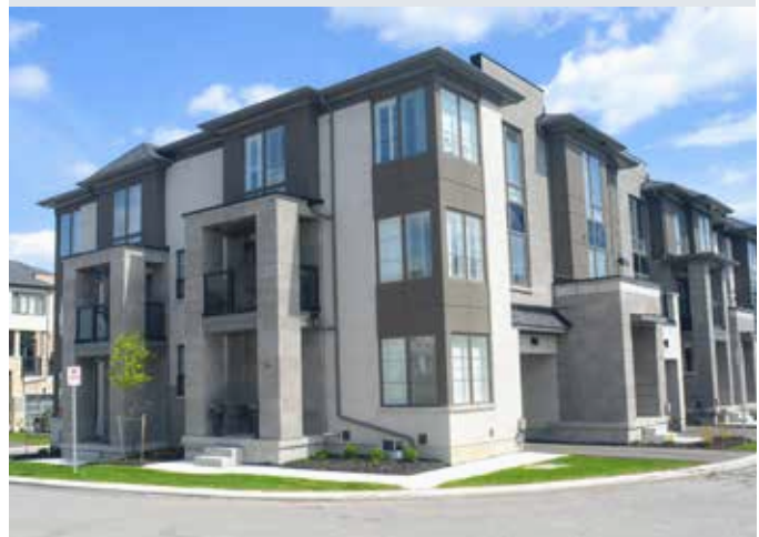
Image example of a back-to-back townhouse with amenity space provided by balconies above the garage.
