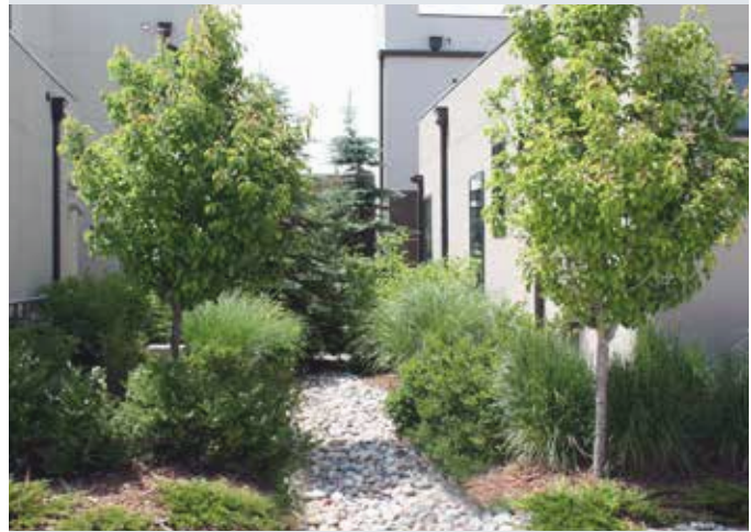
Image example of roof downspouts which help direct excess water into soakaway pits.
