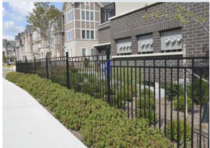
Image example of metal fence, with planting to screen the utility meters from immediate public view.
