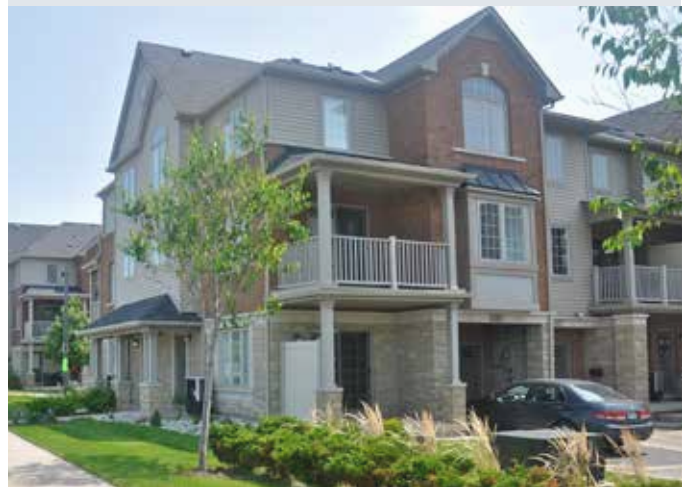
Image example of a back-to-back townhouse with amenity space provided by balconies.
