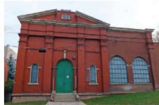
Ferguson Avenue Pumping Station, looking East
