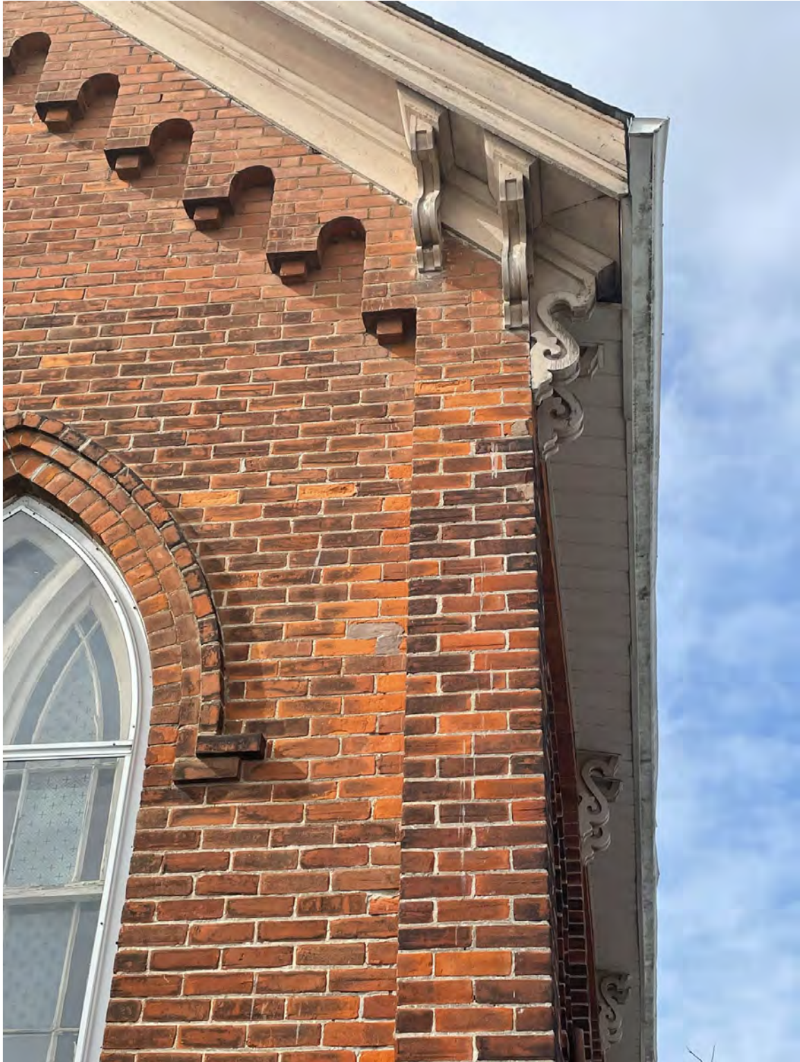
DECORATIVE WOOD BRACKETS, BRICK CORBELLING, SHALLOW BRICK BUTTRESS, & RAISED BRICK HOOD MOULD
