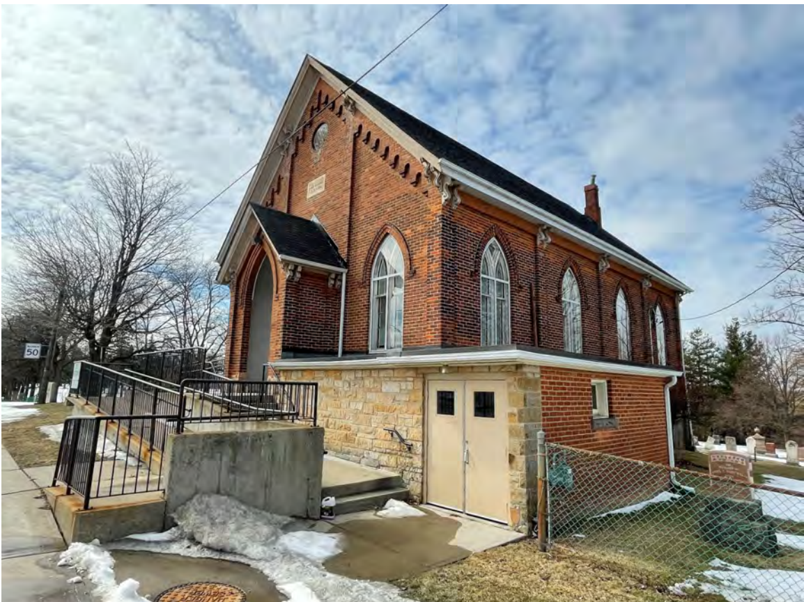
20 TH CENTURY ADDITION – 1-STOREY WITH BRICK AND STONE CLADDING TO MATCH THE CHURCH
