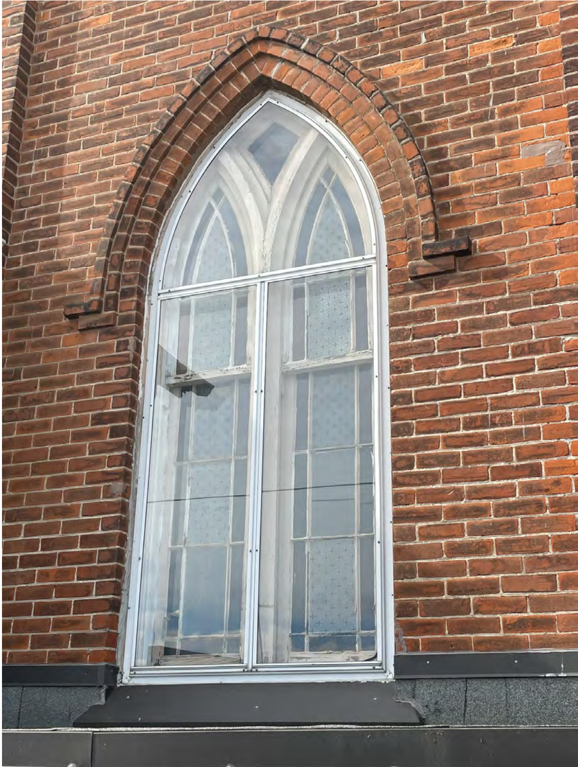
POINTED GOTHIC WINDOWS WITH A RAISED BRICK HOOD MOULD – PAIRED LANCET WINDOW WITH COLOURED GLASS – METAL FRAMED EXTERIOR STORMS INSTALLED
